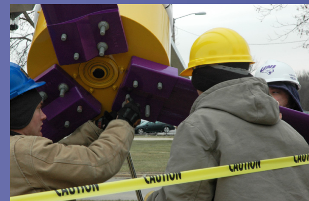
Blade installation to hub
