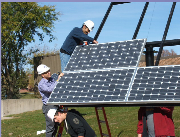
PV panels are installed by students, July 2010
