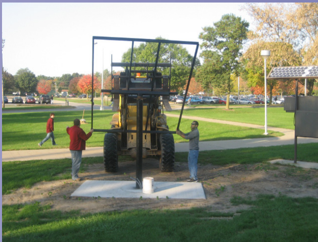
PV panel frame installation, July 2010
