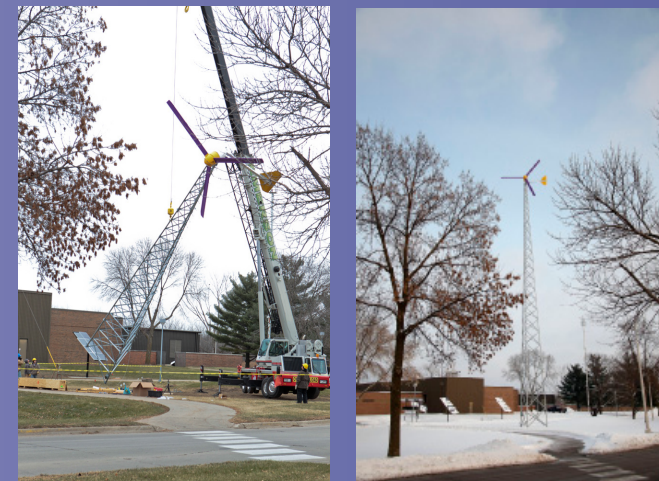
Installation and Final Project
